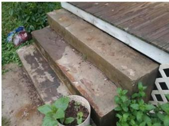
Issue There are cracked steps. This permits water penetration, and will lead to further damage. Location Rear porch
